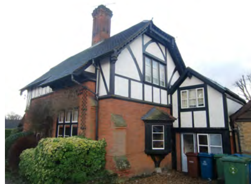
Picture 1.35 View looking south towards 47 West Drive
