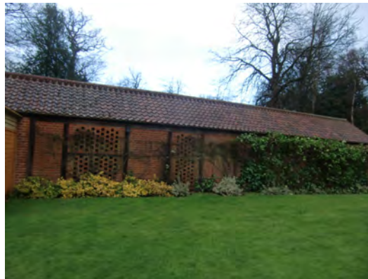
Picture 1.34 Replica drying sheds within the Kiln site, Brookshill re-using original clay pantiles
