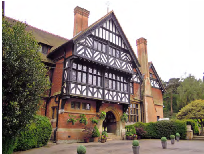
Picture 1.51 Architecture by Norman Shaw
